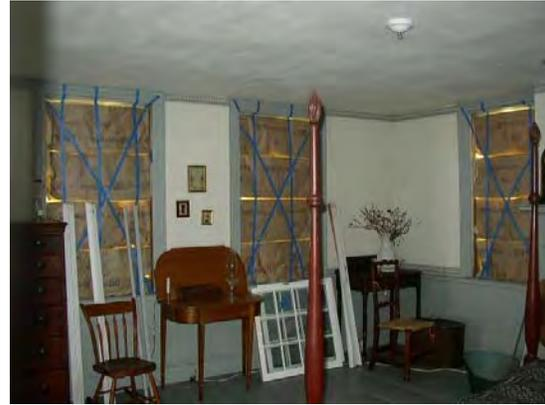
*First floor south room at Thompson House with sashes removed and temporary insulation installed.*
